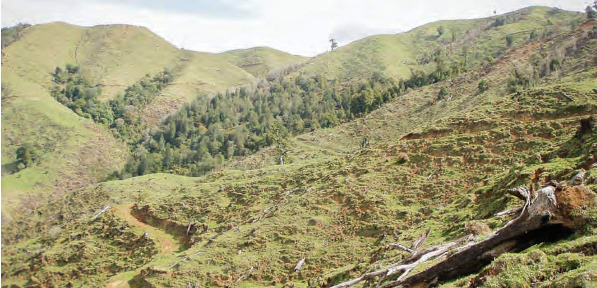
A mixture of high erosion land and remnant vegetation in the Moakurua catchment.
